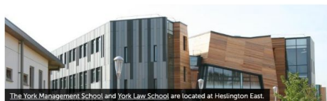
The York Management School and York Law School are located at Heslington East.
